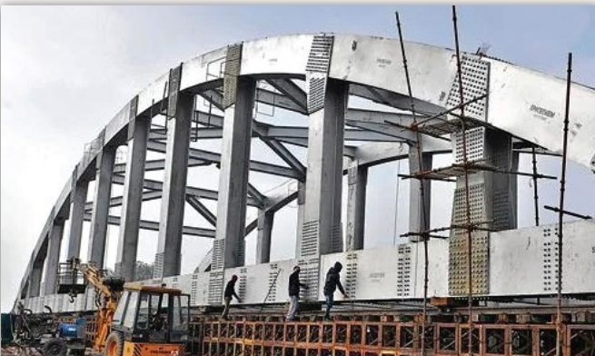
Bow String Bridges
