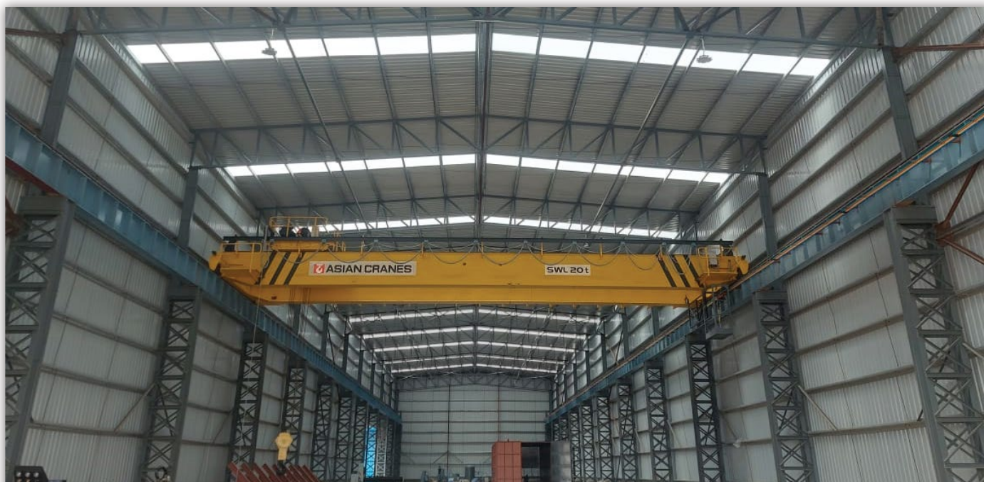
20 tons lifting capacity EOT crane with a clear height of 8 meters
