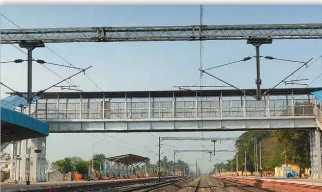
Foot Over Bridge
