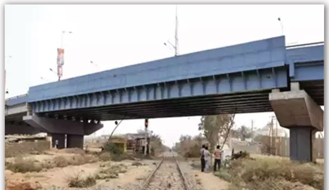
Rail Over Bridge
